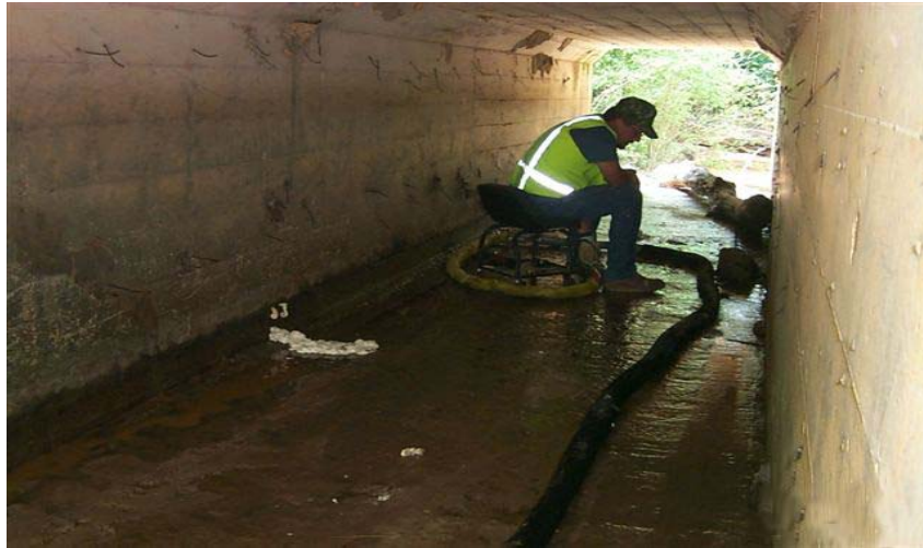
Figure 5 - Injecting Polymer Material into one of the 3-Barrels
