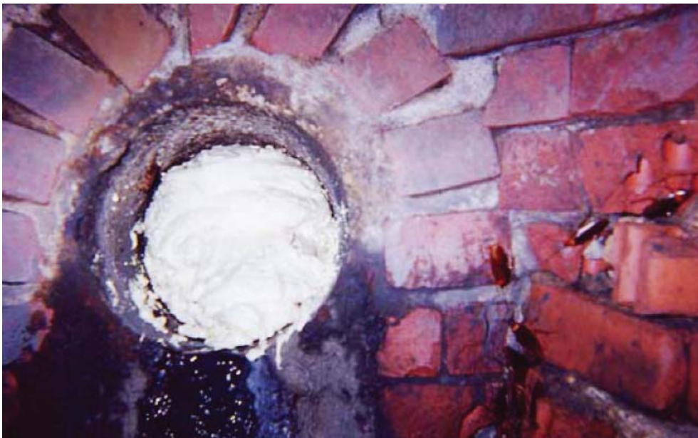
Figure 4 - Sealed 8-inch Sanitary Sewer Line, 25 Feet Below Ground
