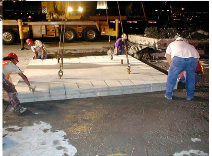
Placing Panels, During Off Hours
