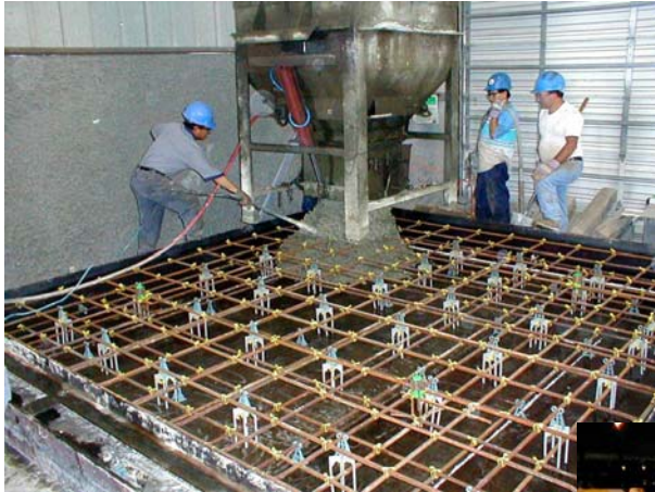
Creating Pre-Cast Panels, Off-Site
