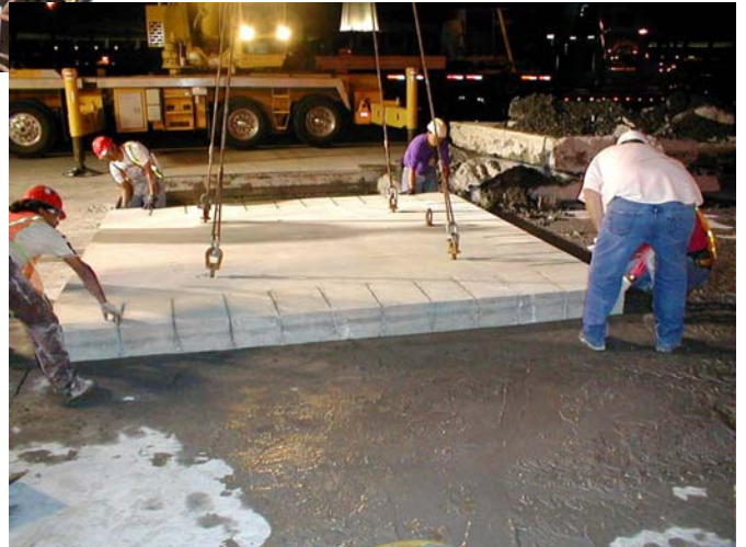
Placing Panels, During Off Hours
