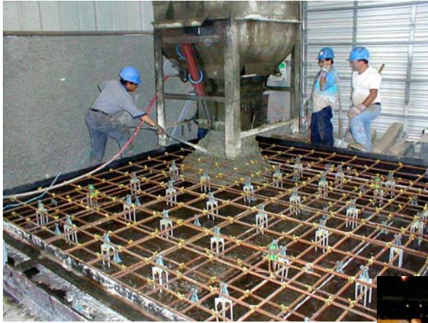
Creating Pre-Cast Panels, Off-Site
