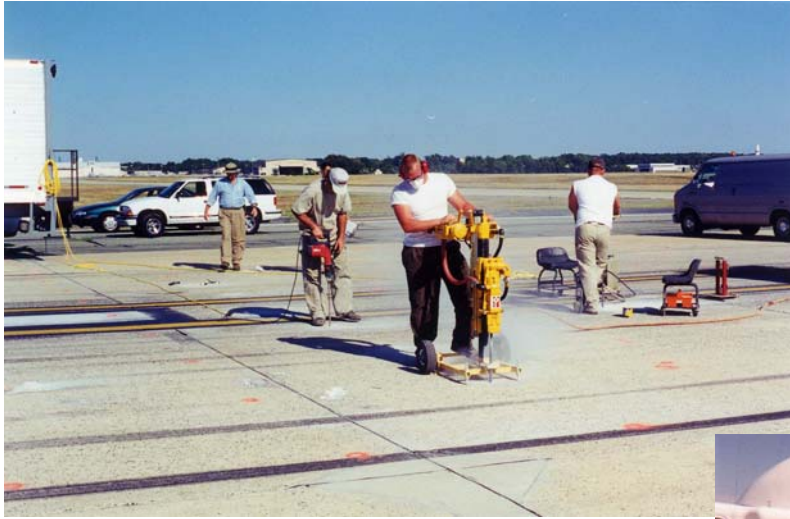
Drilling Injection Holes In Runway
