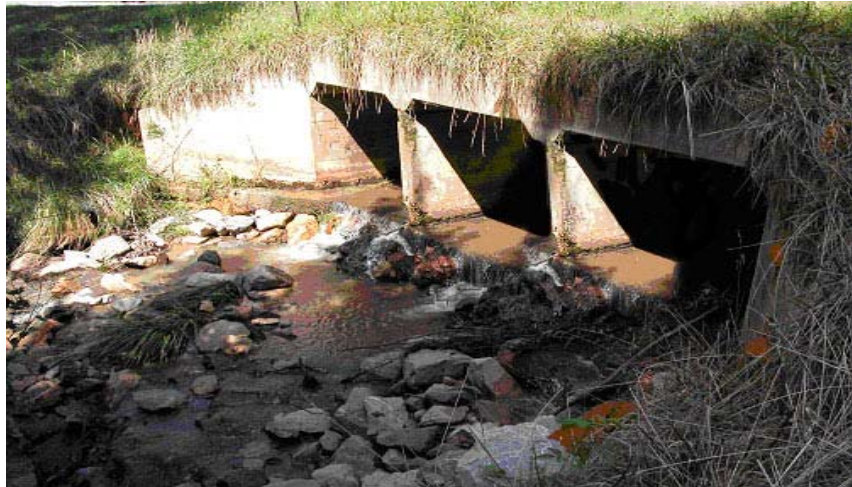
Figure 6 - Water Correctly Exiting Through the Repaired Culvert
